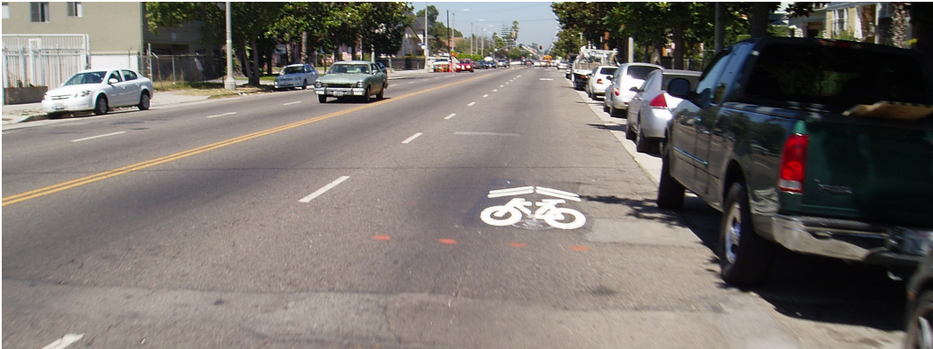
Figure 4 Adams Blvd SLM installation with orange markings to help guide video analysis measurements
