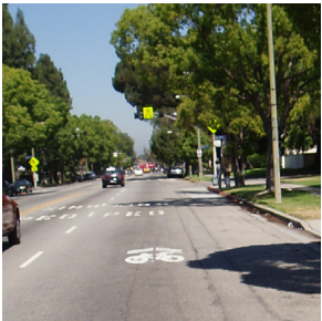
Figure 5 Adams Blvd before (top) and after (bottom) shared lane marking application
